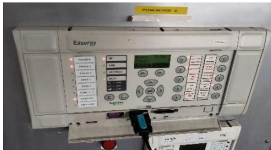
Gambar 12. Relay Distance Gardu Induk Dolopo
