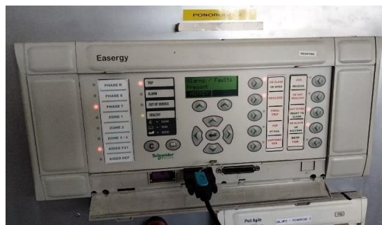
Gambar 20. Relay Distance Gardu Induk Dolopo
